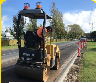
Road upgrades and installation of new loading ramps at the Saleyards.
