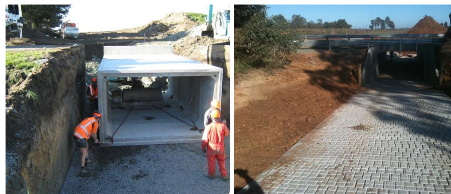
Figure 33 – Construction and completion of cattle underpasses.
